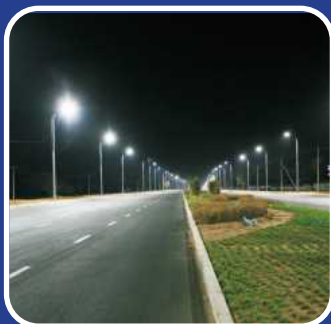
HIGHWAY AND ROADWAY
